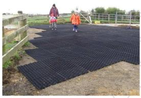
3. The final stages were the filling of the JakMatGeocell with a locally sourced Huntly "Crushed Brown Rock" and then rolling. This particular aggregate was chosen for it soft, crumbling characteristics which allowed it to compact tightly into the cells of the mat as well as be sympathetic to the cow's hooves. This layer was to approximately 20-40mm above the top of the mat on completion.
